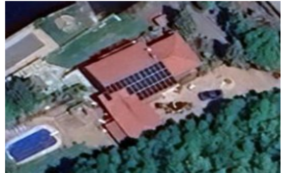
SITE AERIAL VIEW
